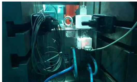
Fig. 22 Installation of edge device
